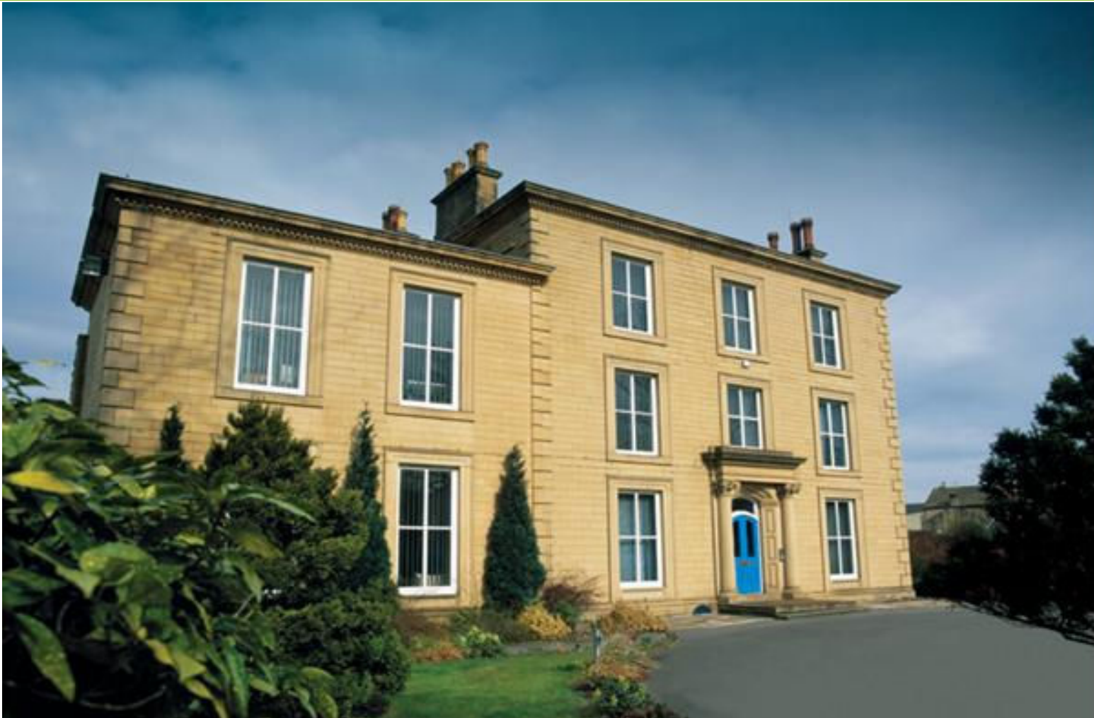
Leigh House, Varley Street, Pudsey, Leeds, LS28 6AN
